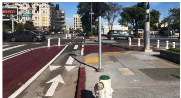
A Quick-build curb extensions in Oakland near the Lake Merritt BART Station.
